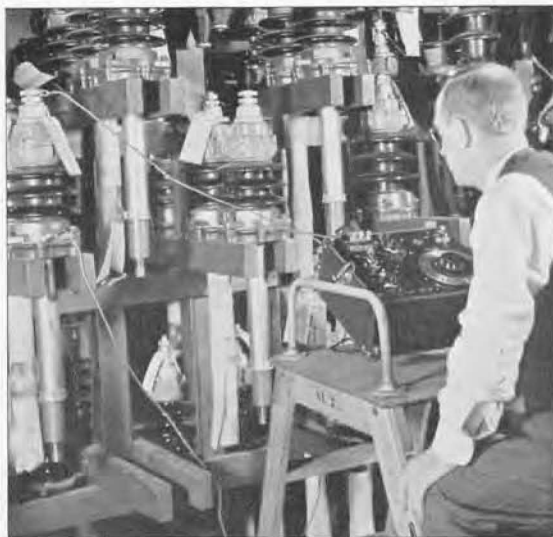
Measuring bushings on a storage rack with the TYPE 740-BG Capacitance Test Bridge.
