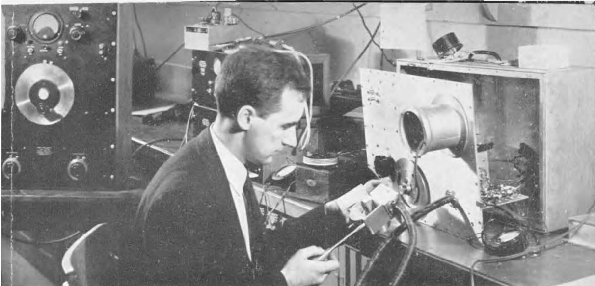
Above—Development work on an experimental standard-signal generator.
