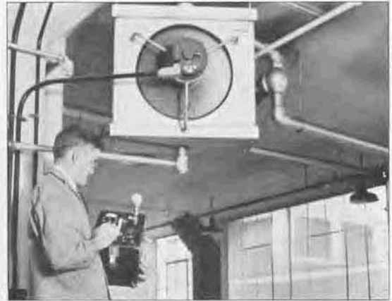
Measuring the noise from a ventilating fan with the sound-level meter.
