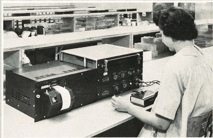
1680-A Automatic Capacitance Bridge Assembly used to make high-reliability quality-control tests. Measurement results are visible immediately to the operator and are recorded by the 1137 Data Printer. Photograph courtesy of Erie Technological Products, Inc.
