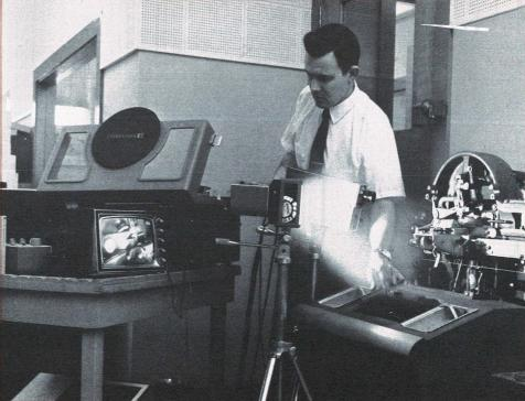
Its brightness and versatility make this strobe a natural for TV applications such as video recordings of rapidly-moving parts in mechanical devices.
